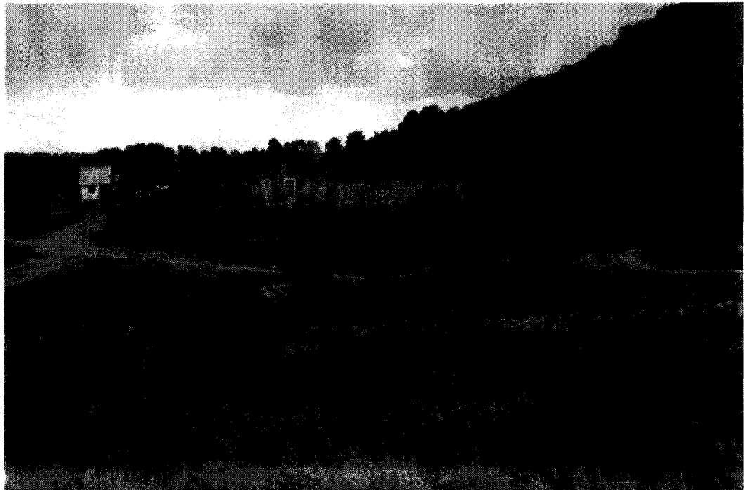
Photo 4. Looking to the west boundary of the Site. Residential dwellings can be observed adjacent north to the Site.
